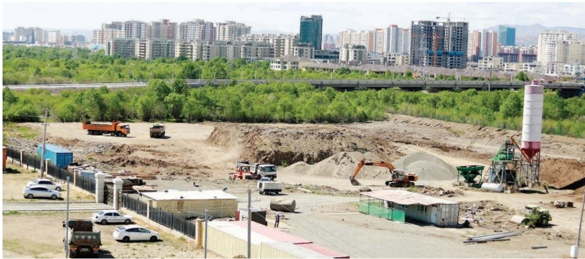
Figure 4. Floodplain erosion of Tuul River
