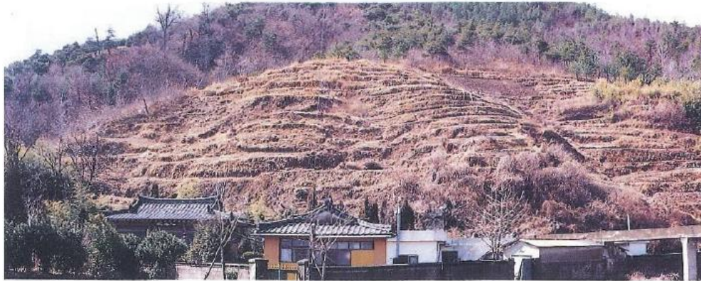
Before preventive erosion control
